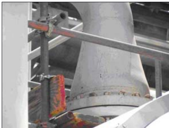
Fig. 1a (left) shows a general view of the selected 20-in. x 12-in. reducer; Fig. 1b shows the fiber-optic sensors attached on the reducer.
